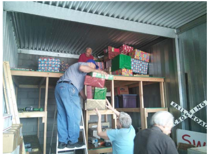
8' legs were attached to the existing shelves along with the framework to support the new floor
