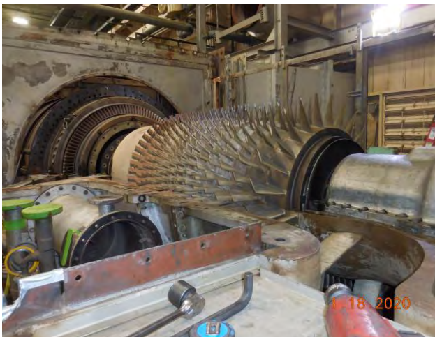
With the case removed you can see the old turbine about to be removed
