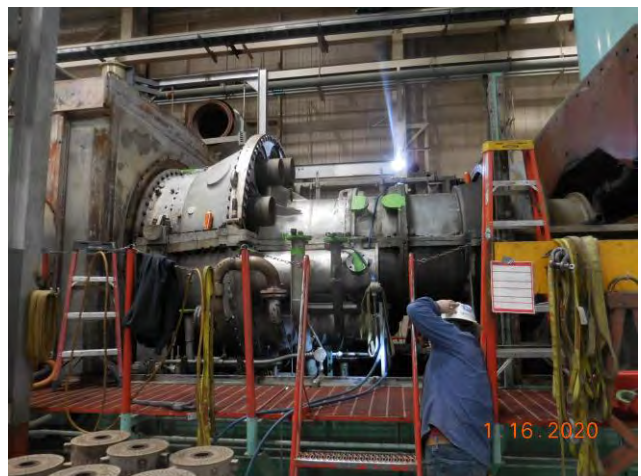
With the maintenance "skins" removed you can see the turbine with the horizontal split case
